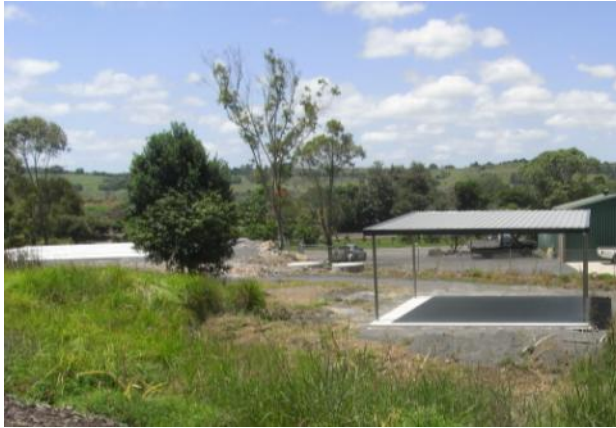
Environmental Education Centre and Water Management Pavilion under construction
